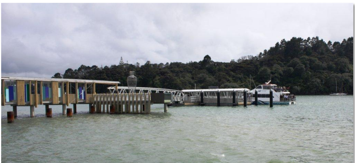
Figure 5: Completed Hobsonville Ferry Wharf
