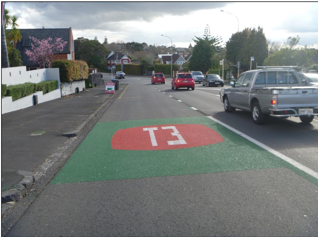
Figure 1: New trial T3 lane marking on Remuera Road
