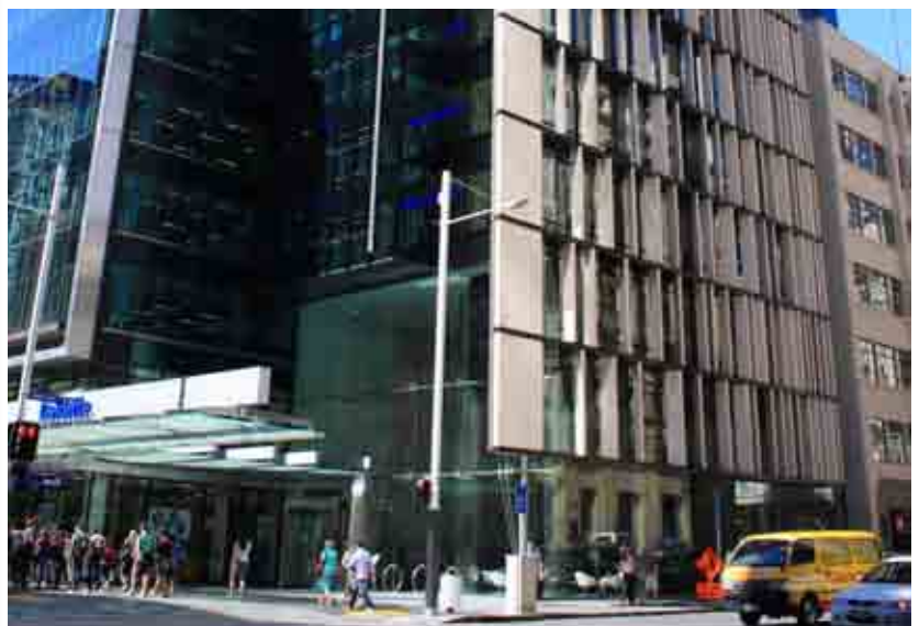
Standards for high quality and sustainable business accommodation will provide a competitive advantage for businesses with a high level of environmental ethos
