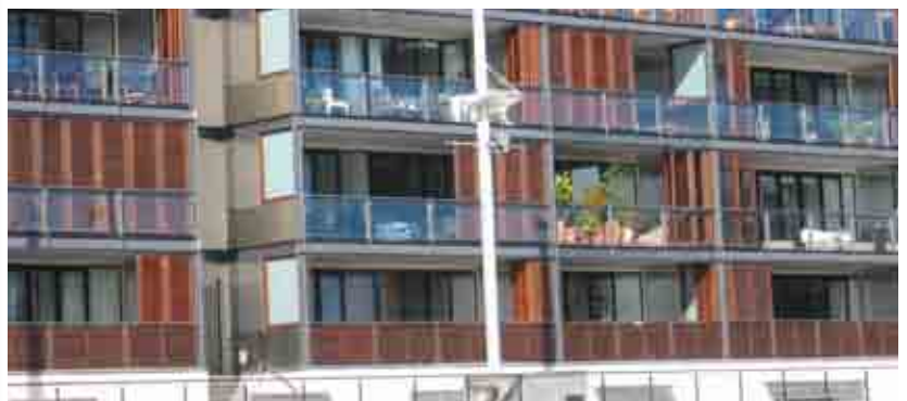
Better standards for residential accommodation encourage a more positive response to higher density living.
