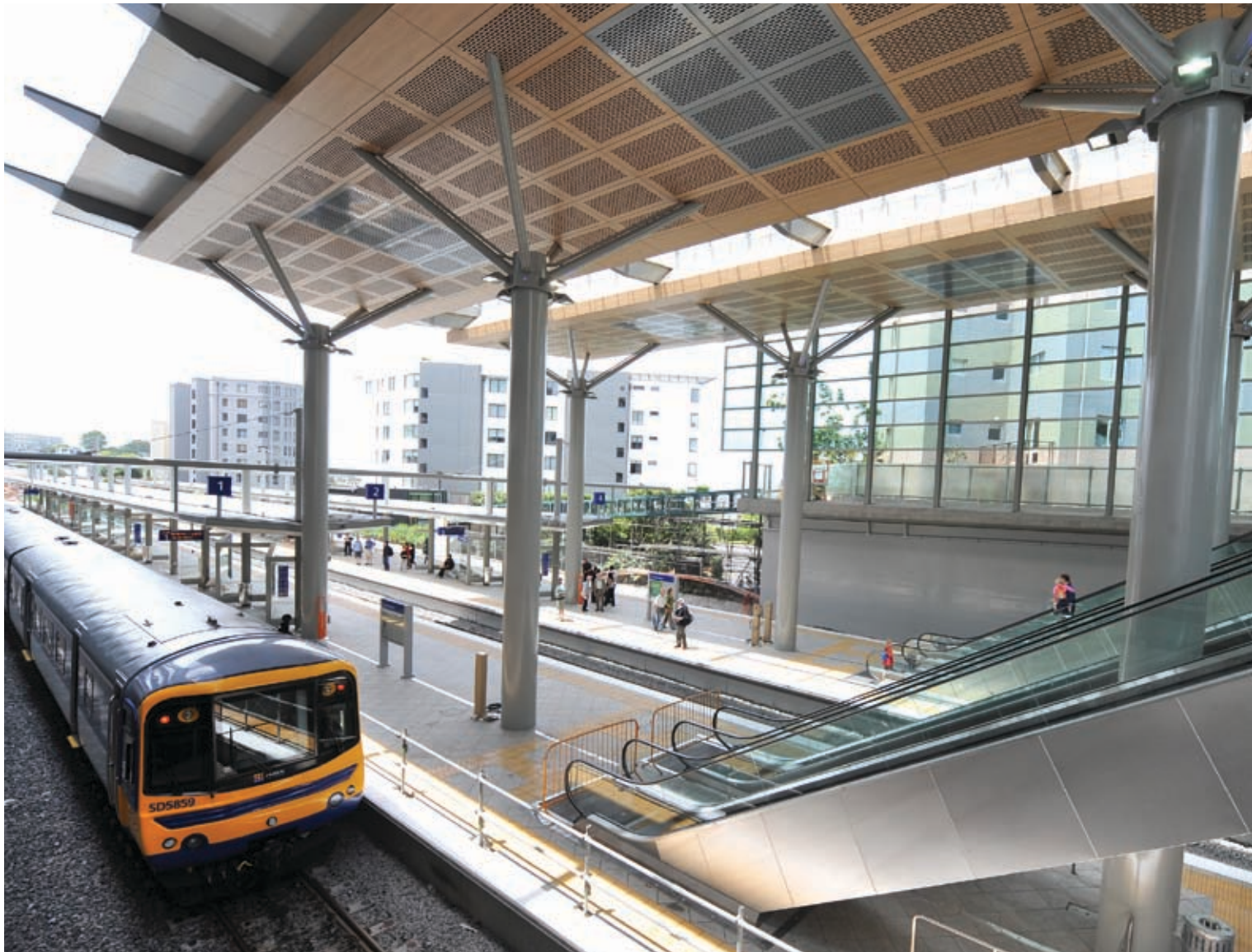
Newmarket Station upgrade, showing off its sleek lines and high tech design, in preparation for the new electric trains and electrification of the main trunk line, as well as the anticipated increase in passenger numbers in the coming years.
