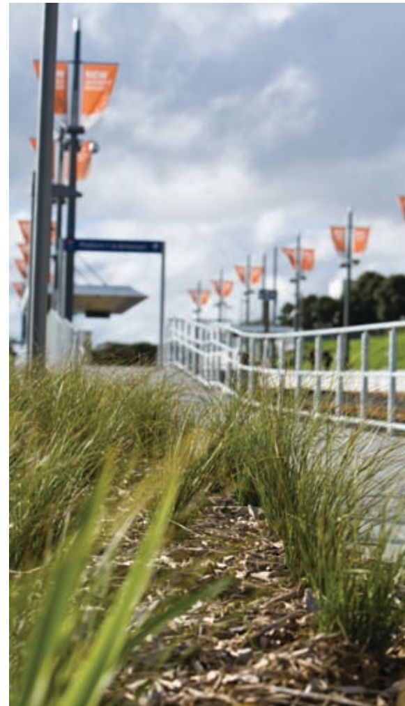
When it was Avondale Station's turn to be upgraded, the new design included relocating the station to better fit with Auckland City's redevelopment plan for the town centre. The station opened in June 2010 and its above-platform facilities cost $1.6 million.
