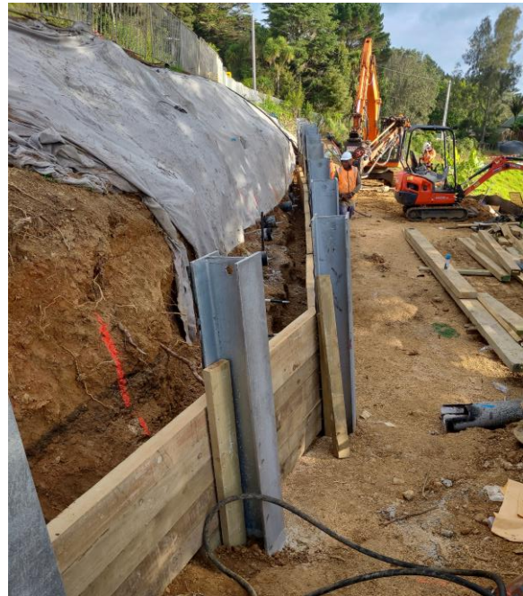
First stage timber lagging being installed.
