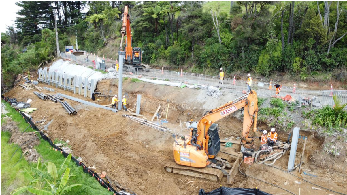
Piling and anchoring work starting on second stage.
