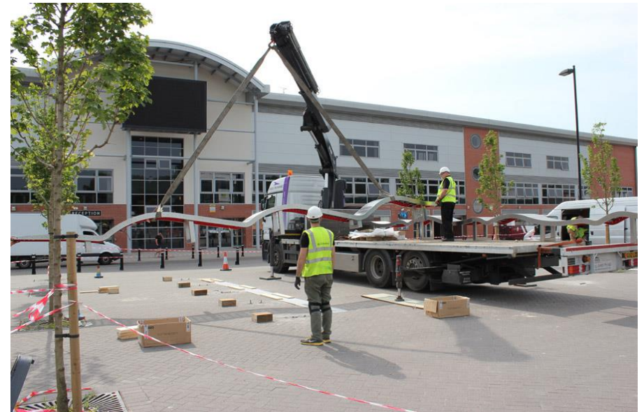
Example of a HIAB lifting operation.
