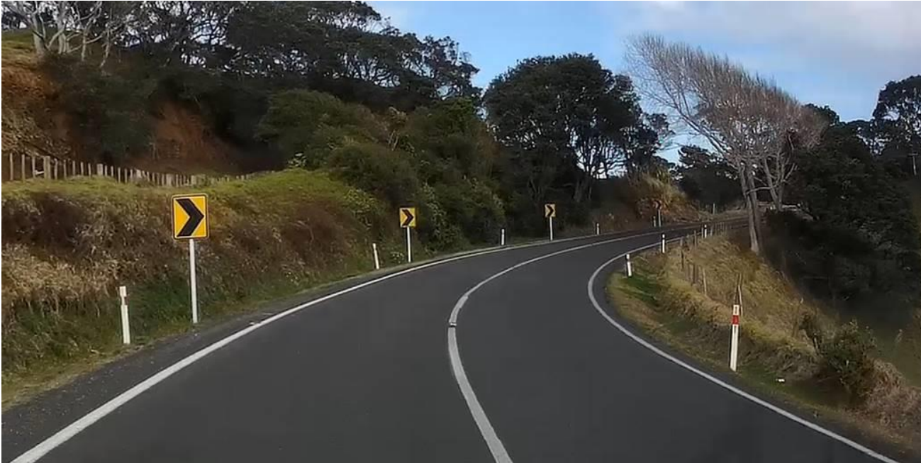
Awhitu Road, Waiuku with recently installed safety chevron signs.
