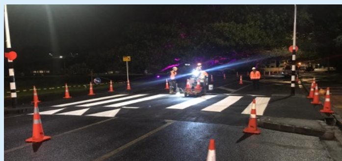
The finishing touches being put on the new raised pedestrian table on Tamaki Drive, which was finished on Tuesday night.
