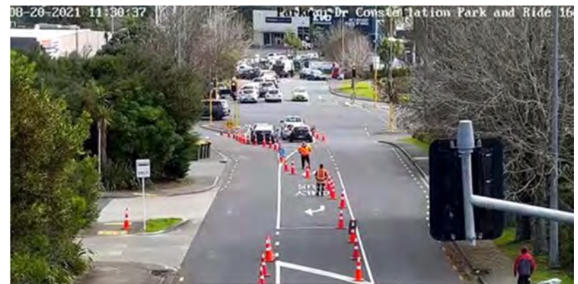
Figure 2 20 August 2021 | Intersection of Parkway Drive & Constellation Drive, Rosedale before and after detours
