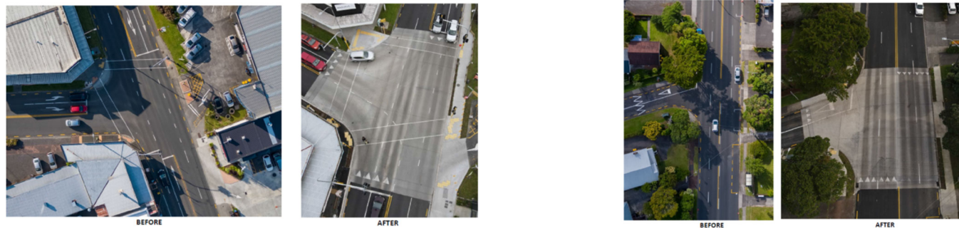
Figure 2 Raised intersections at Glen Eden Town Centre
