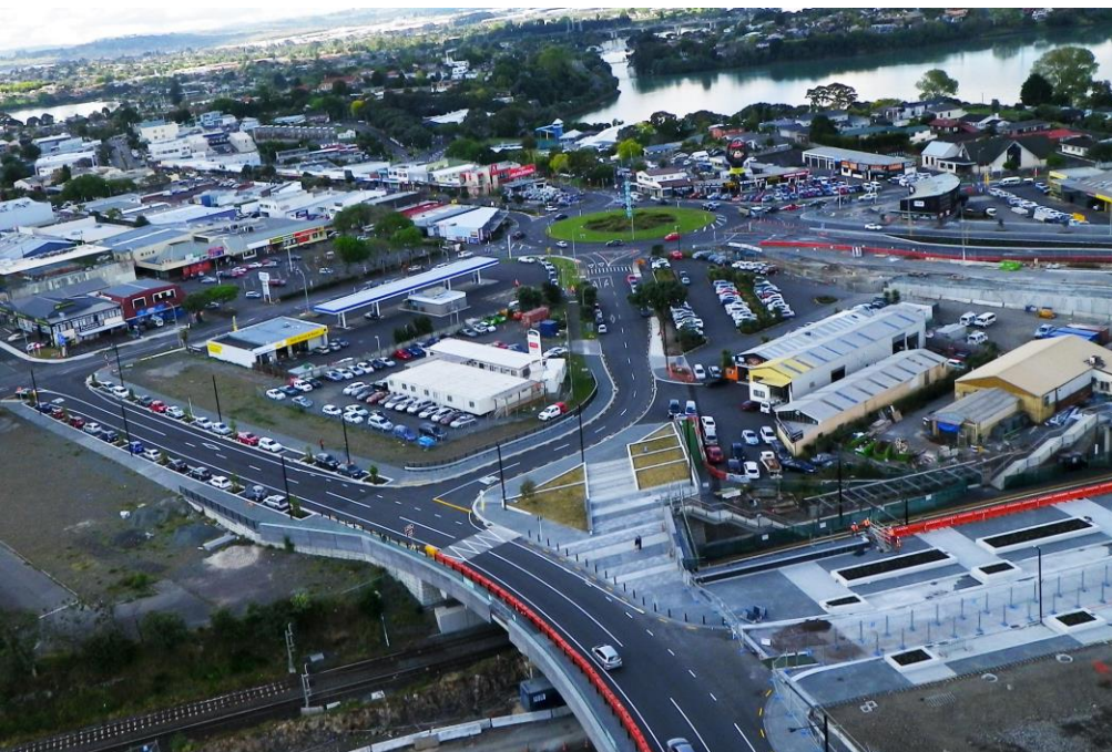
Mountain Rd Bridge
