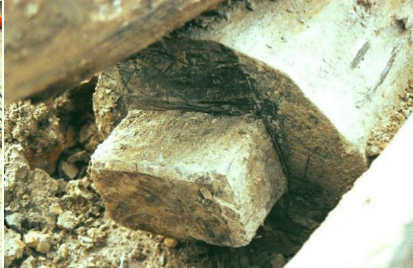
Queen St jetty piles – detail of tenon dressing
