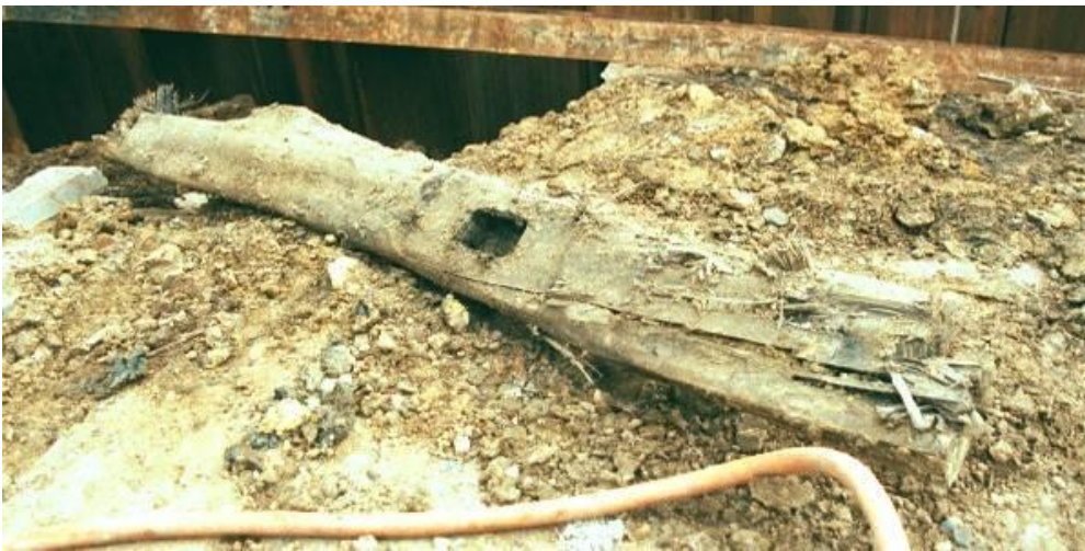
Queen St jetty pile showing mortise
