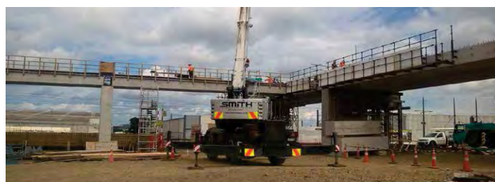
Photographs of the concourse beams being lifted in
