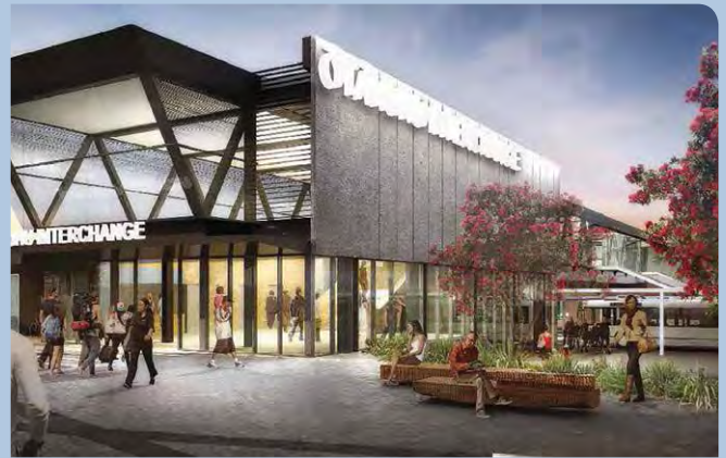
Plaza area in front of Interchange entrance
