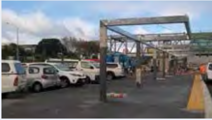
Installation of steel frames for bus platforms shelters / canopies.
