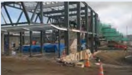
Ticket hall & amenity building taking shape; view westward along the concourse.
