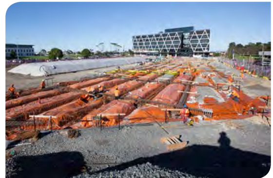
Installation of foundation reinforcing
