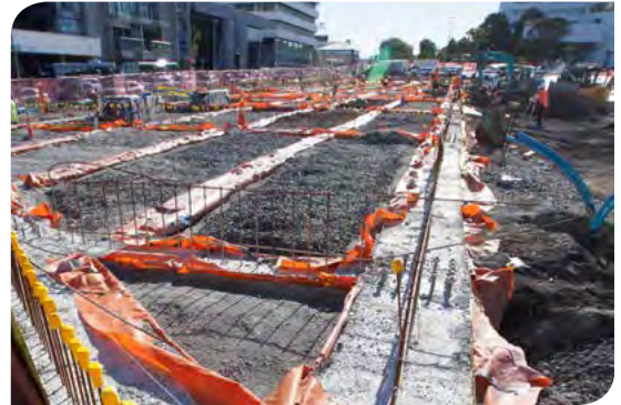
Ready now for erecting steel work at the western end
