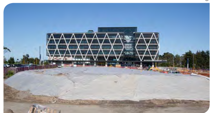
Relocated preload on top of the future bus operation area
