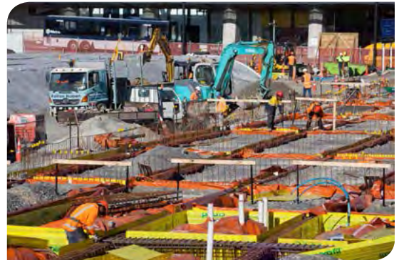
Installing and tying foundation reinforcing
