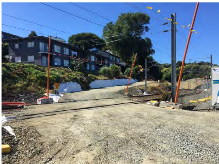
Temporary access road across tracks to Western Abutment
