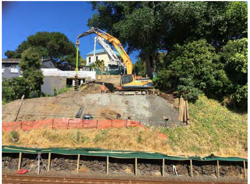
Auger drilling holes for temporary pole retaining wall at bottom of Cowie St
