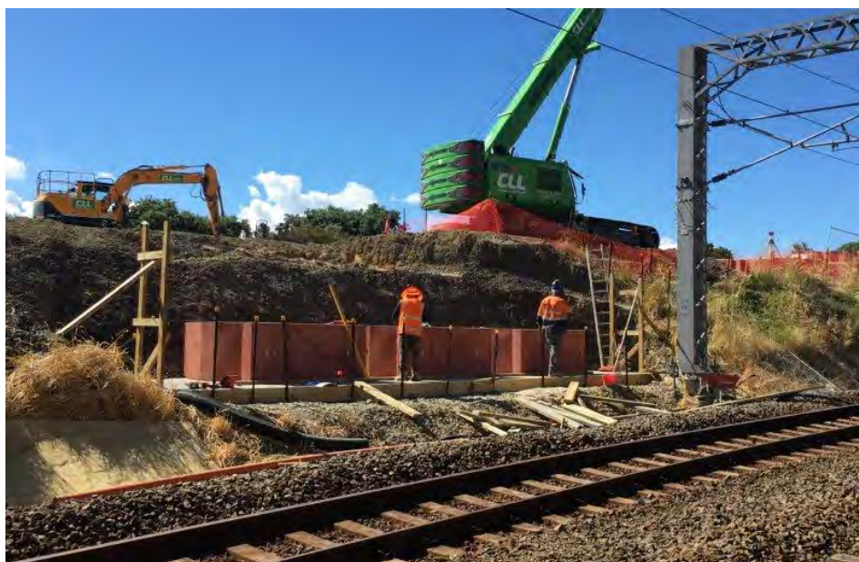
Eastern Abutment first layer of blocks in place
