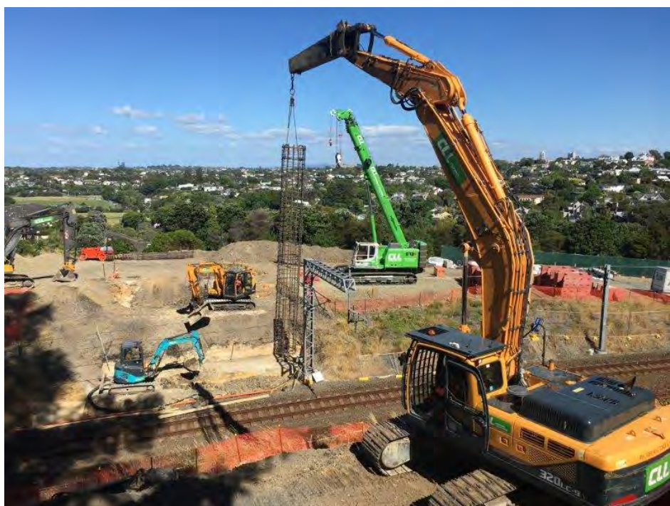
Reinforcing cage for temporary piles on Western Abutment
