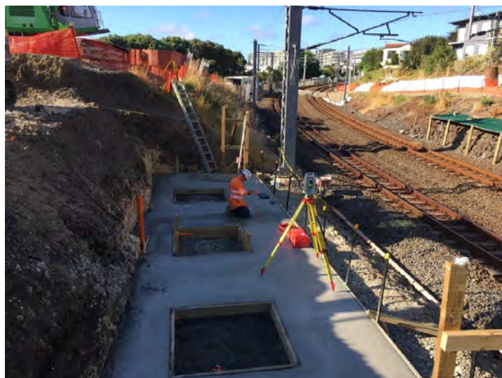
Foundation prepared for front of Eastern Abutment
