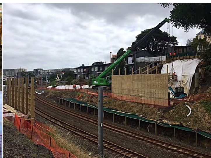
Timber separation hoardings (Western Abutment on right)
