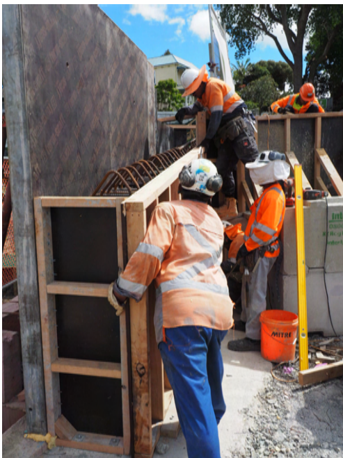
Boxing for a wingwall
