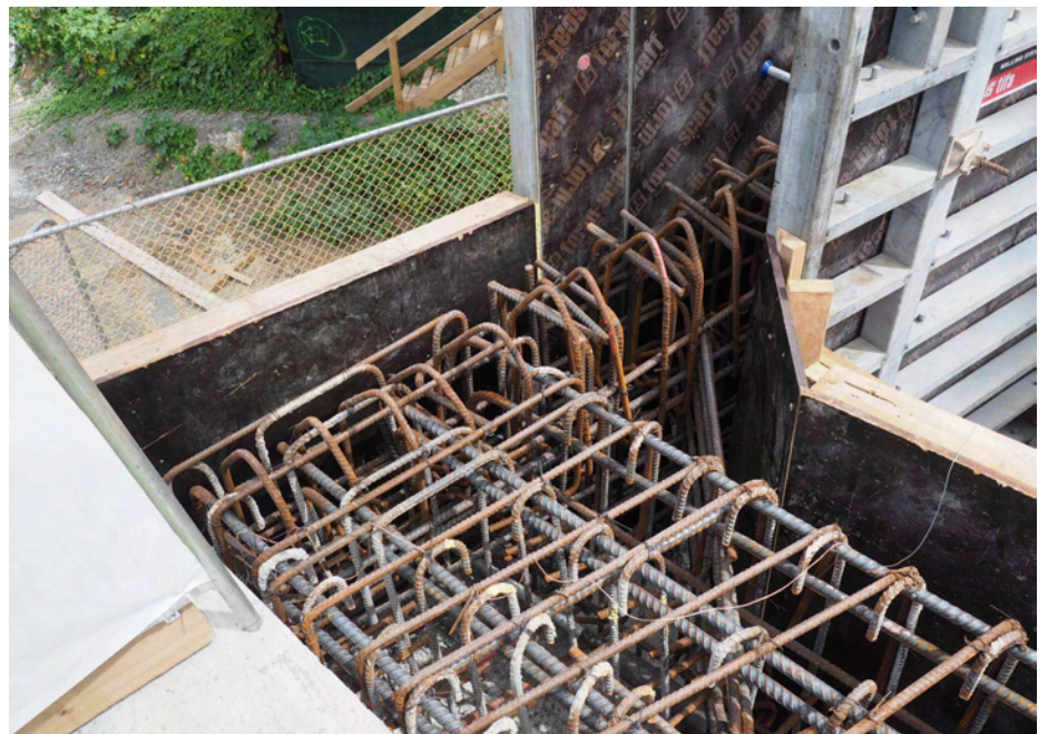
Reinforcing in headstock (front) and wingwall
