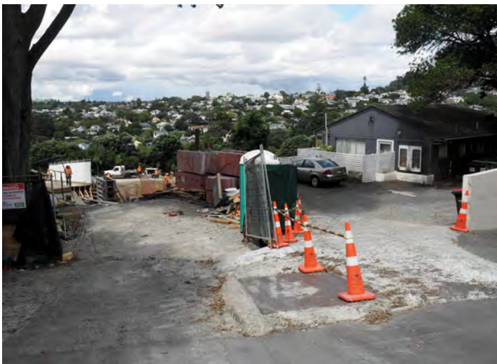
Concrete pad for removal
