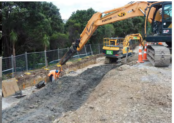
Inserting mesh for piles on retaining wall
