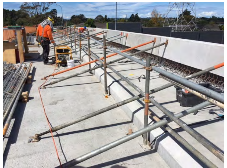
Example barrier and footpath
