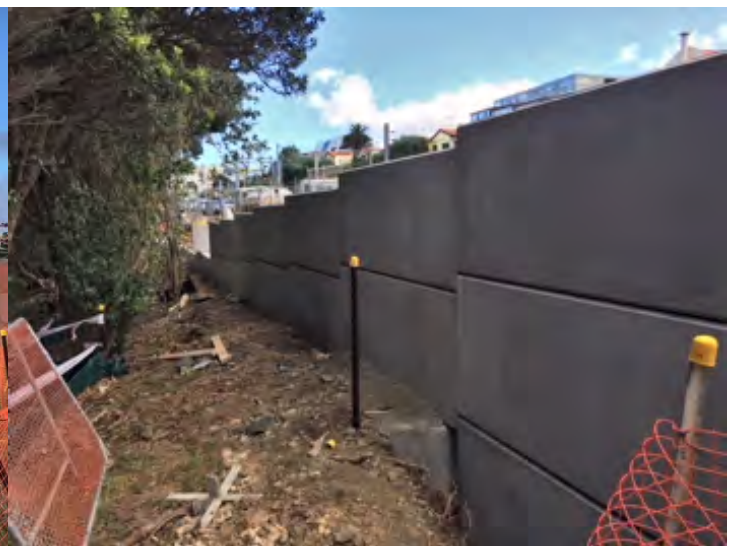
Front face of new Laxon Terrace retaining wall
