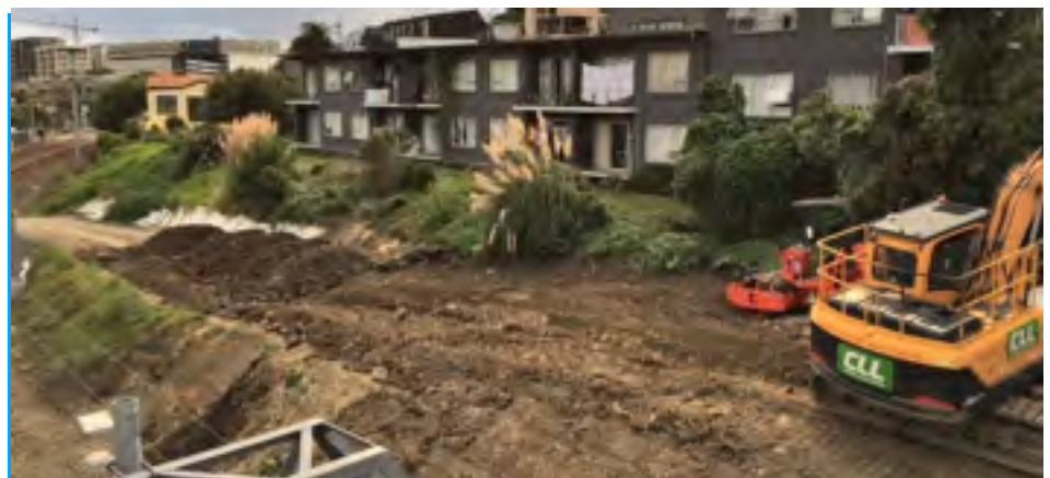
Reinstating the bank below 9 Cowie Street
