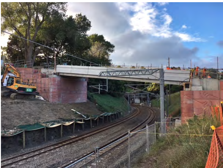
The precast bridge barrier in place
