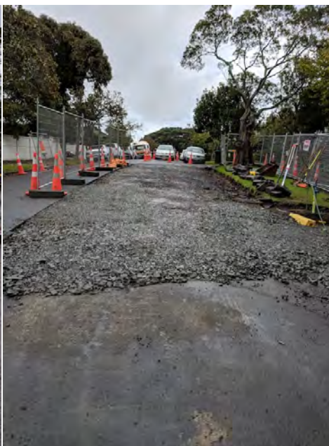
Start on road formation
