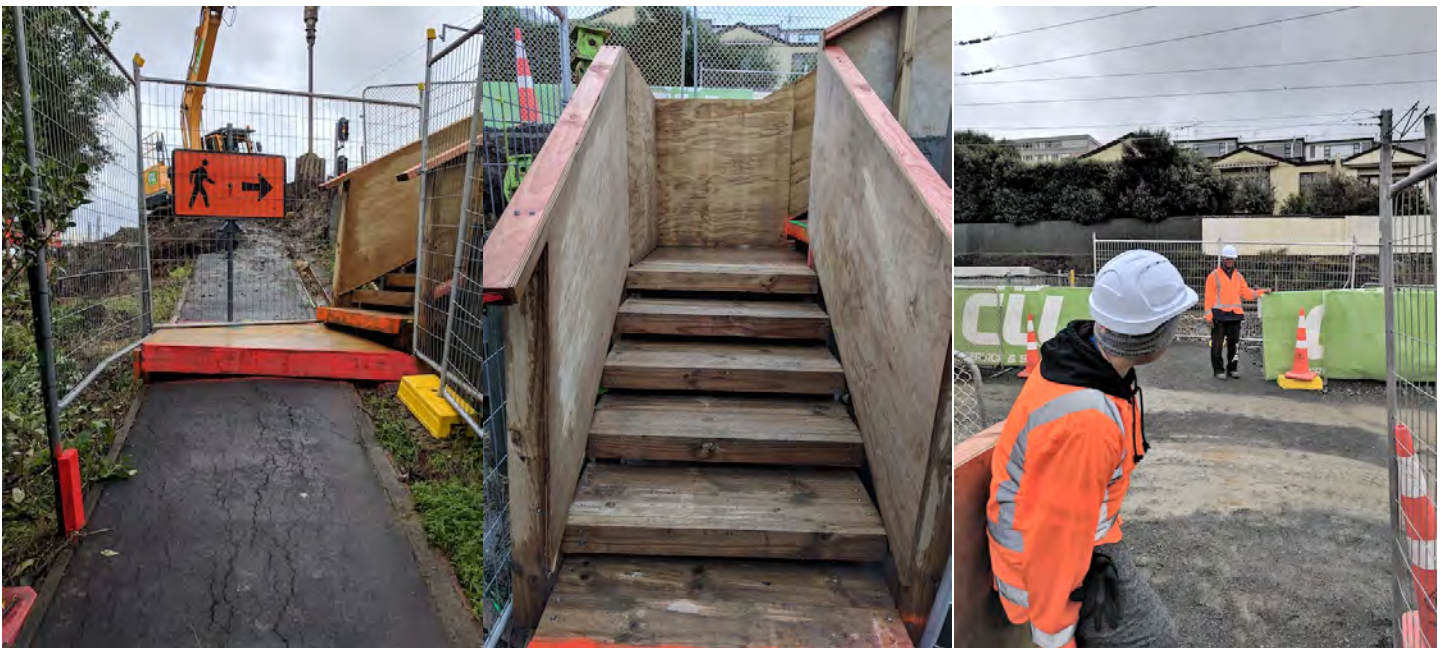
Temporary access route at top of footpath into Newmarket Park
