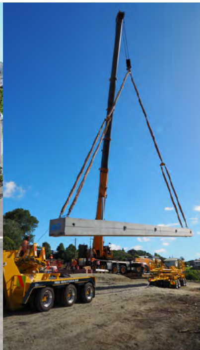
Craning into position of one of the beams
