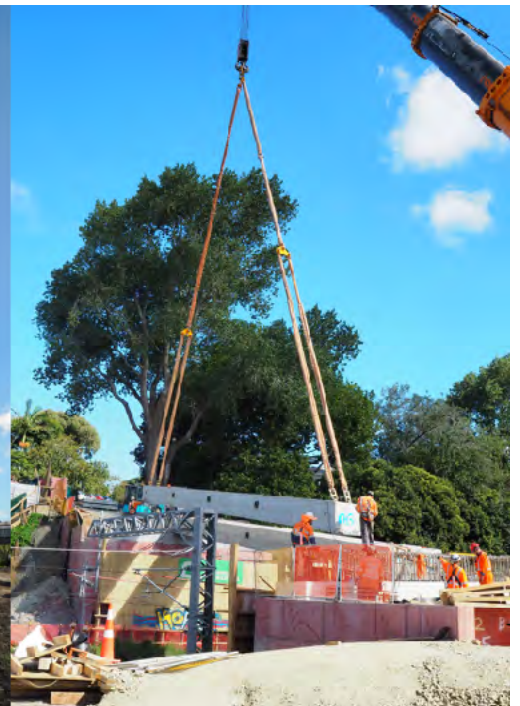
Craning into position of one of the beams
