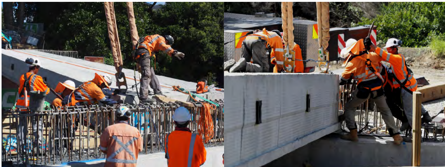
Final positioning of one of the beams
