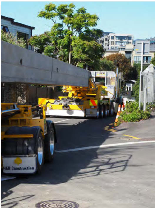
Reversing into the site from Laxon Terrace
