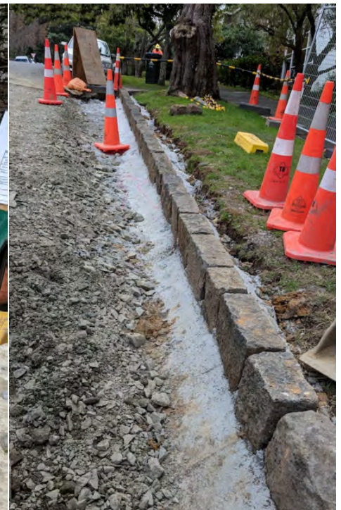
Bluestone kerbing in Cowie Street
