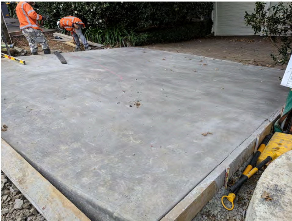
Replacement vehicle crossing at 6 Cowie Street
