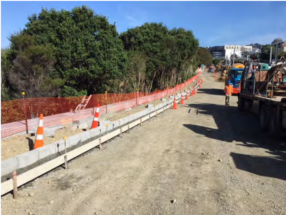
First kerb and channel in new section of Laxon Terrace
