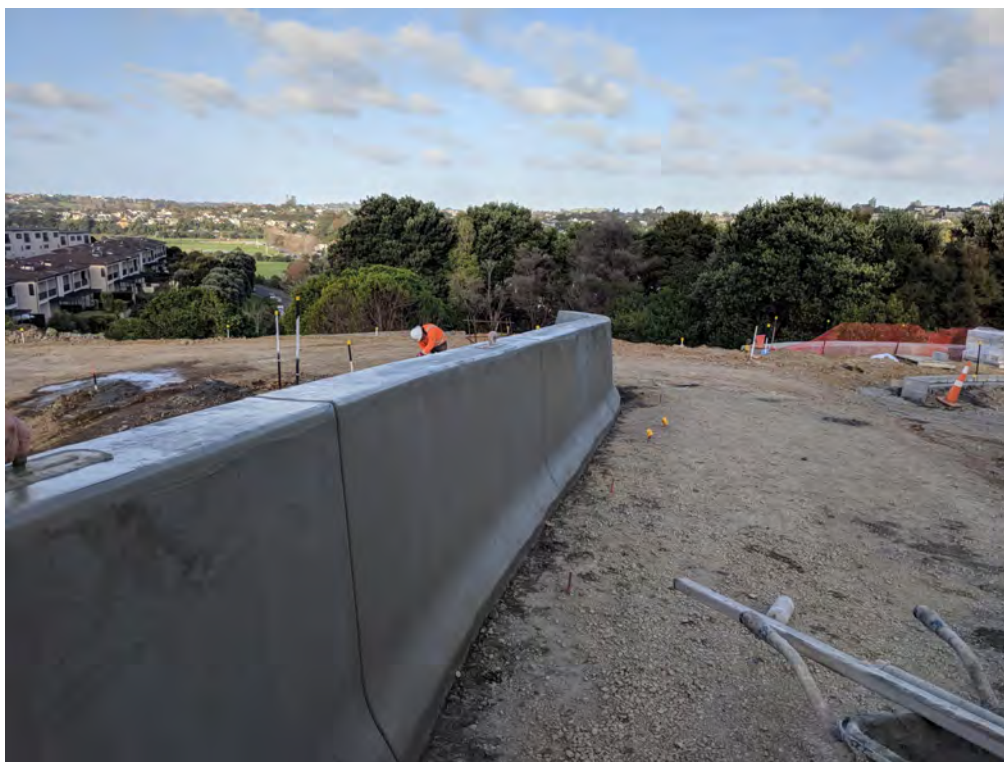
Slip-formed concrete barriers on the approach to the eastern bridge abutment
