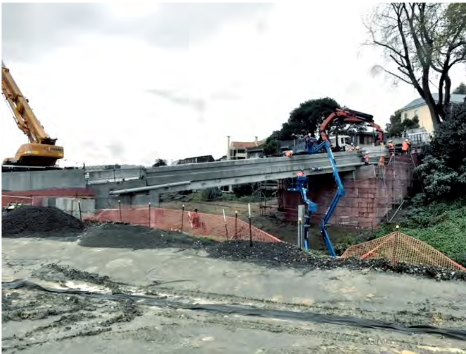
Stormwater pipe being installed on side of bridge
