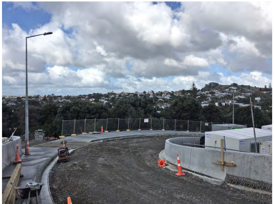
Bridge getting close to completion
