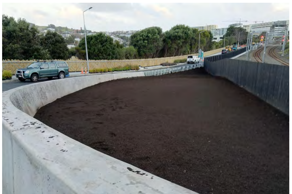
Area at corner next to the bridge ready for planting
