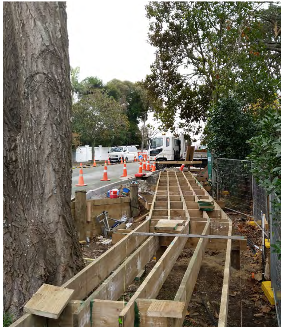
Boardwalk under construction around the poplar tree in Cowie Street
