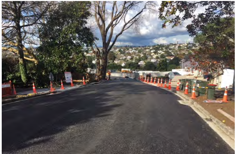
Asphaltting complete on lower Cowie Street
