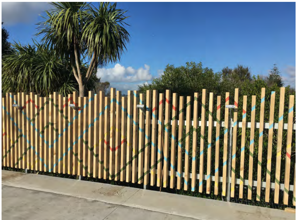
Mana Whenua fence under construction along new section of Laxon Terrace
