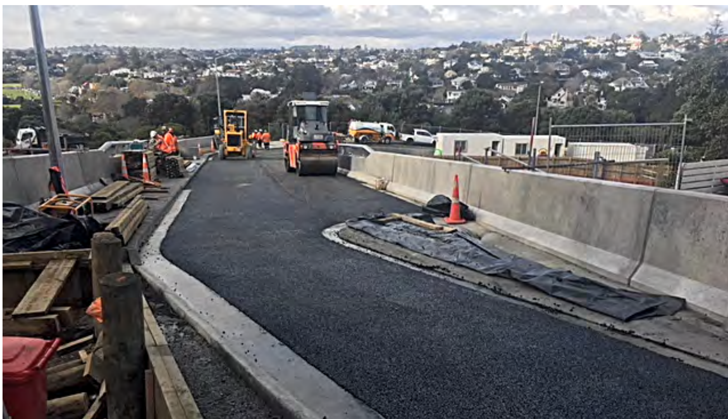
Asphalting the bridge with chicane in foreground
