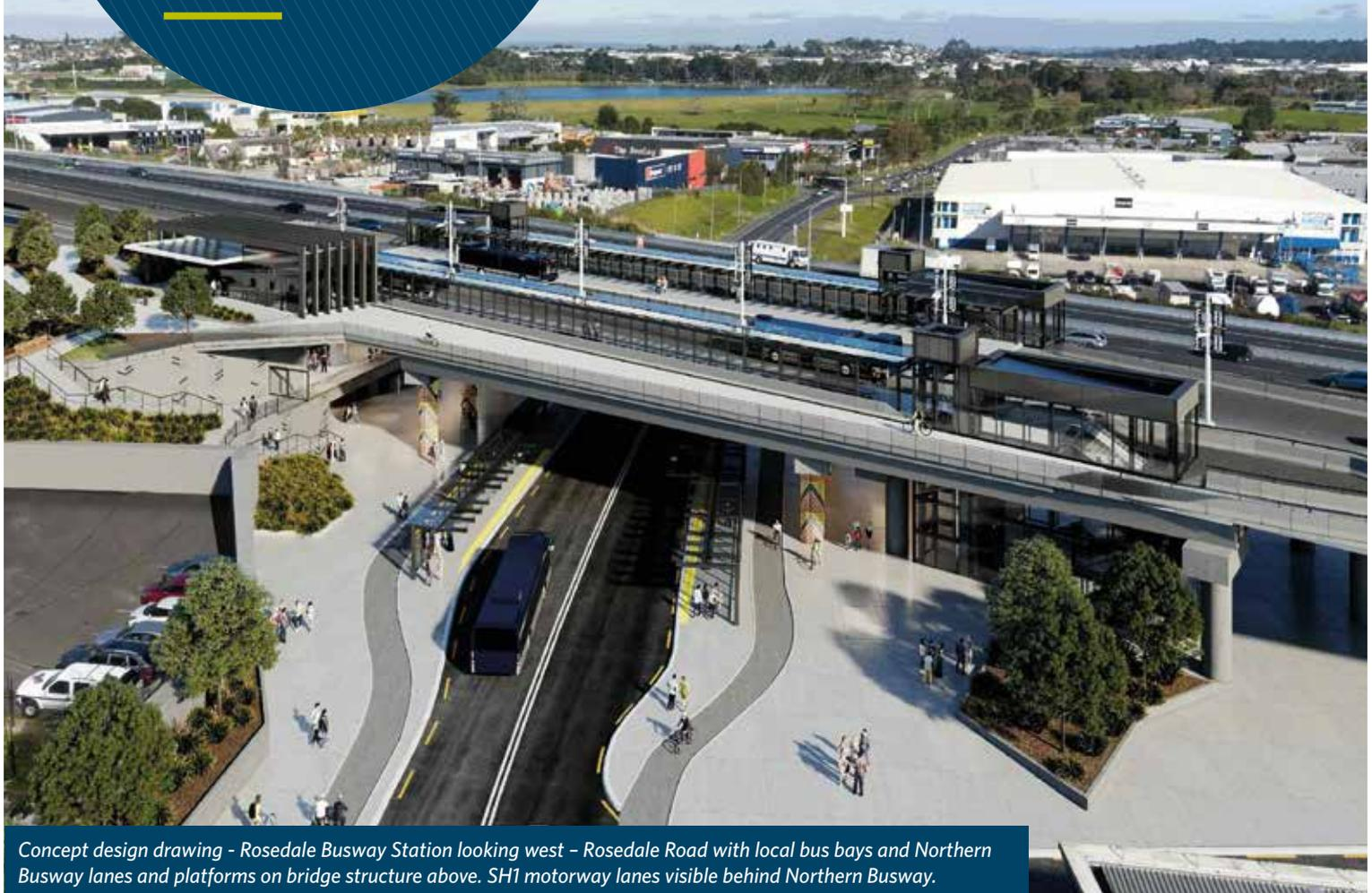
*Concept design drawing - Rosedale Busway Station looking west - Rosedale Road with local bus bays and Northern Busway lanes and platforms on bridge structure above. SH1 motorway lanes visible behind Northern Busway.*
