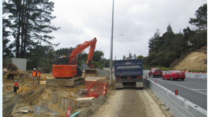
Construction of roundabout retaining walls
