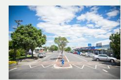
Where pedestrian activity is low, a flush entry threshold with colour or paving difference may be more appropriate, with a calming feature between 6 and 40 m from the intersection continuity line.
