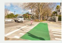
Raised tables may be interpreted by pedestrians as formal pedestrian crossings. This can lead to unsafe use of the crossing point, as pedestrians assume they have right of way. To avoid this, such uncontrolled crossing points should be constructed from a material of an appearance and colour clearly distinguishable from the footpath.
