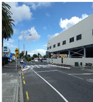
Figure 2 Completed raised zebra crossing at Kolmar Road, Papatoetoe
