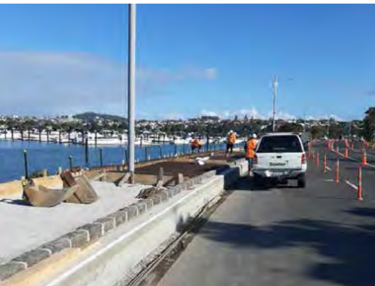
AT has raised the height of the Tamaki Drive seawall to improve resilience to sea level rises
