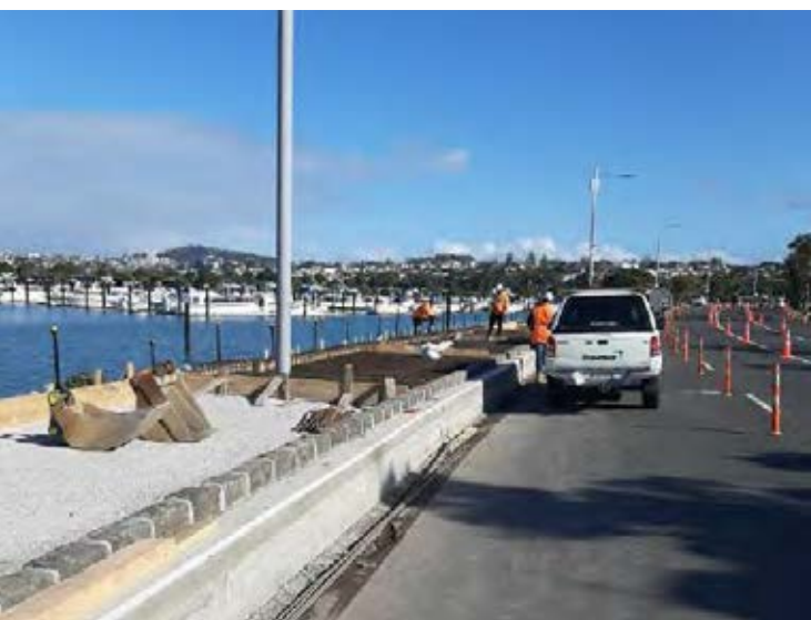
AT has raised the height of the Tāmaki Drive seawall to improve resilience to sea level rises
