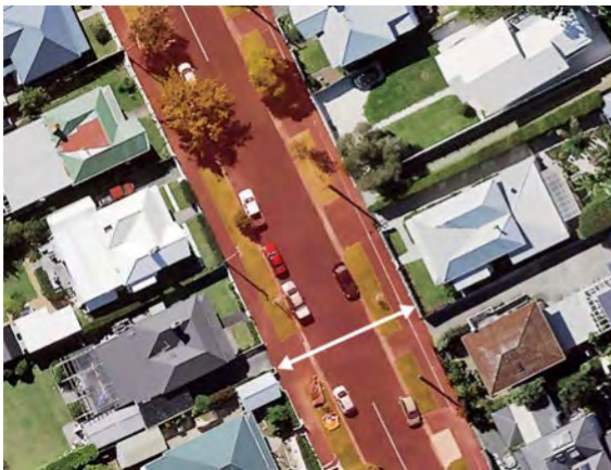
Figure 1: Photo of the road corridor (formed, aerial view)
