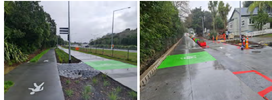
The upgraded North-western Dual Path
