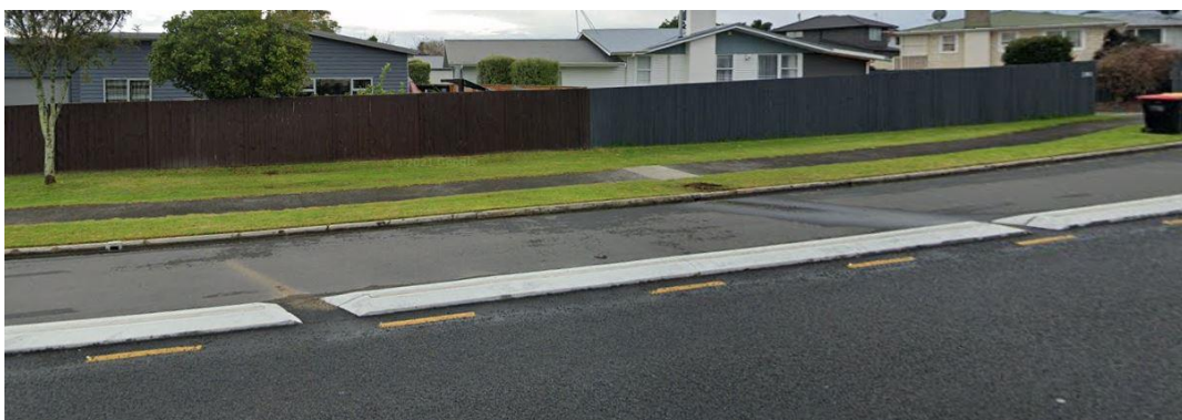
Picture of Embedded Concrete Separators
