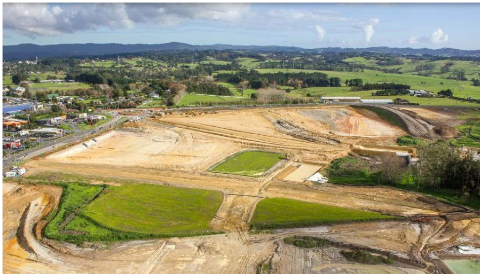
Figure 1: Precinct C Bulk Earthworks
