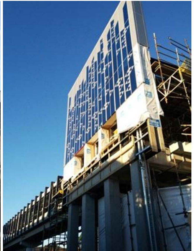
Back of the concourse wall
