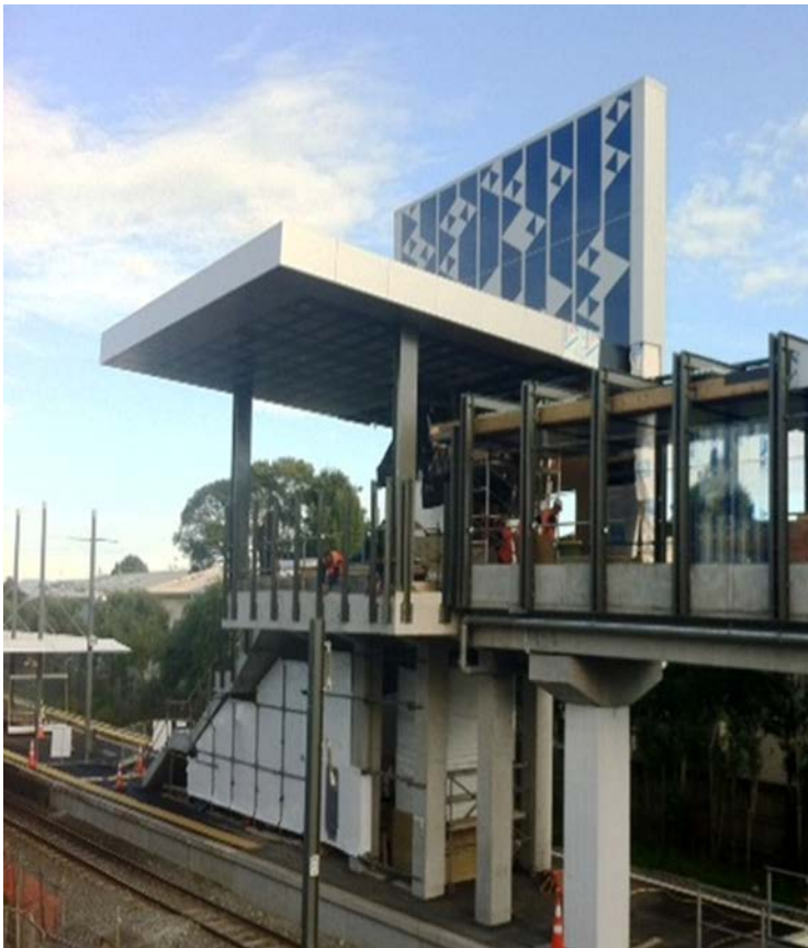
Front of the concourse wall
