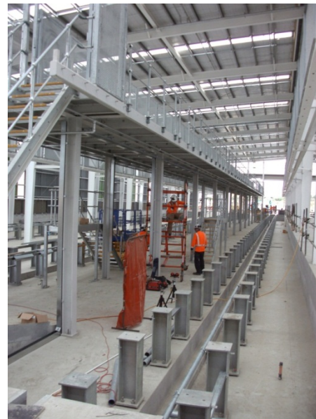
Fig 3: The overhead walkway is well advanced
