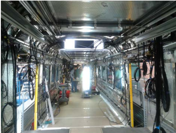
Fig 5: Vehicle being wired. Floors and windows installed
