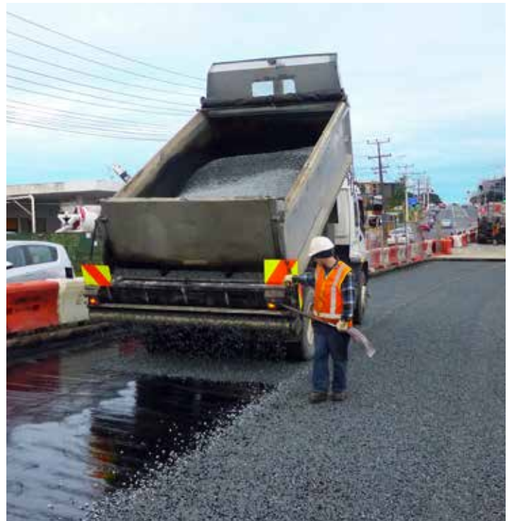
Laying new chipseal on the northbound approach to the bridge
