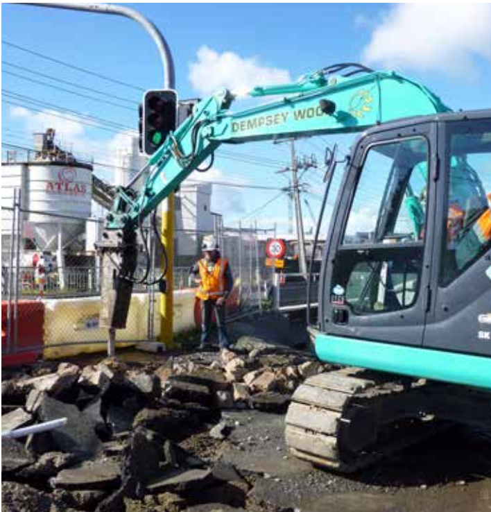
Removing the old road surface on Wairau Road
