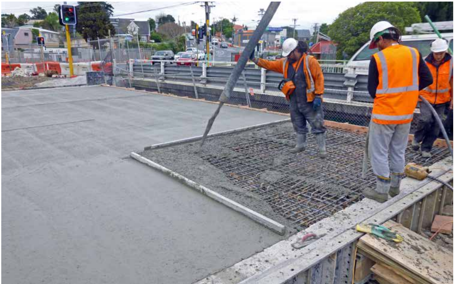
Pumping concrete for the new bridge deck
