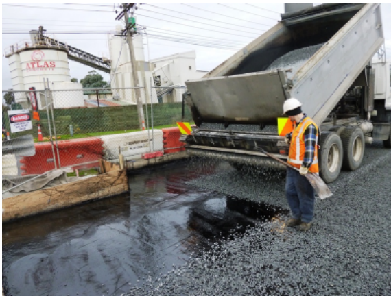
Laying the chip seal on the approach to the bridge
