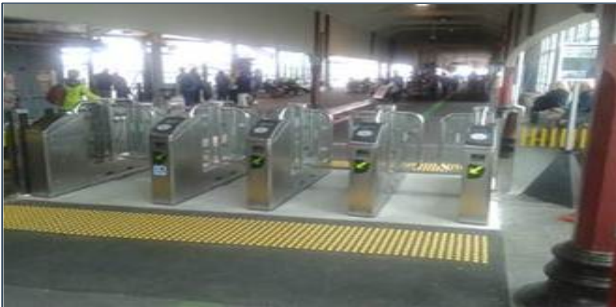
Pier 1 electronic AT HOP gates installed
