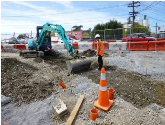
Carrying out kerb and footpath preparation on Forrest Hill Road
