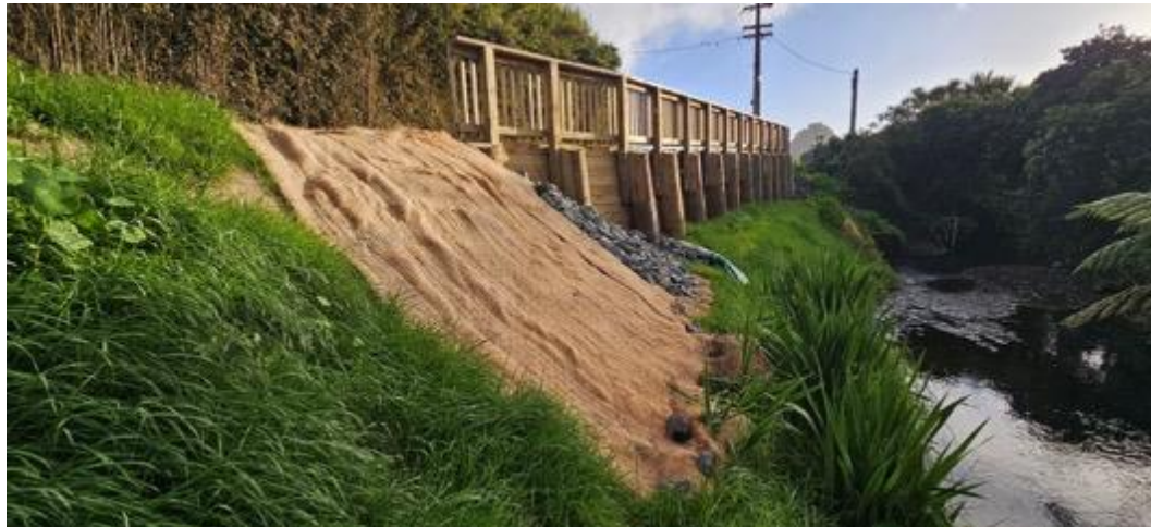
Slip repair on Glenesk Road
