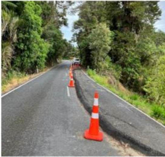
Site ready to start works in early November. The 3D model of the repair shows the slip path and the repair design, which retains the road and pins it back.
