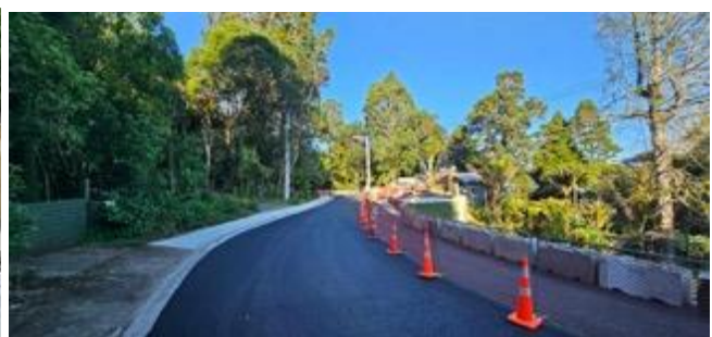
Block retaining wall almost completed on Takahe Road, Road sealed 30 September 2024.
