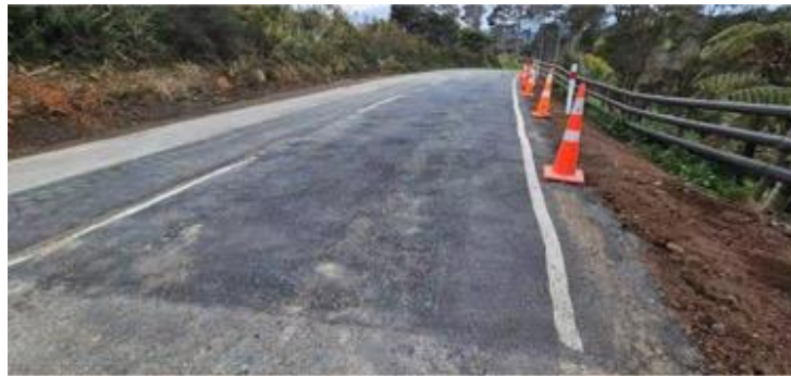
Repaired pavement on Wairere Road, at Roster Ridge.
