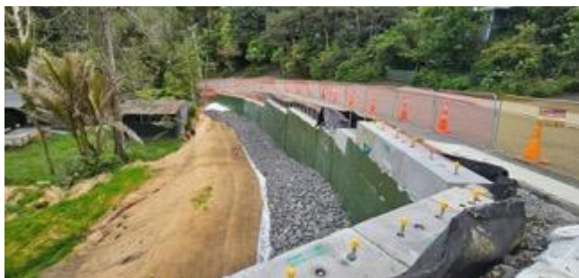
Block retaining wall almost completed on Takahe Road, Road sealed 30 September 2024.
