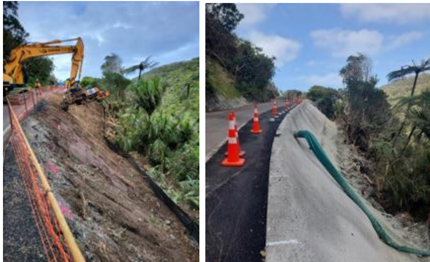
Site underway on Karekare Road, Karekare
