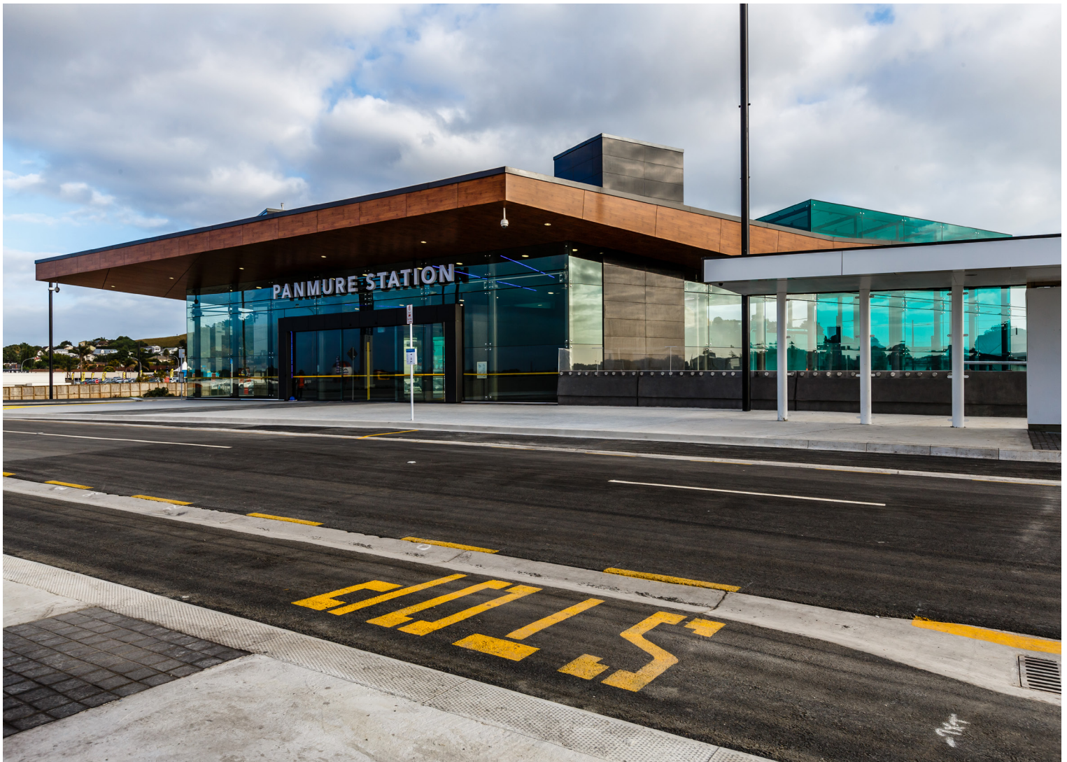
The new Panmure Interchange which was opened in January by Auckland Mayor Len Brown.
