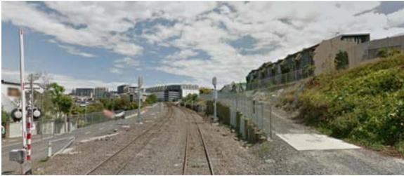
Fig 2 – View South from level crossing. Underpass and road extension proposed to be located between embankment and KiwiRail retaining wall on the right. Underpass road surface would be 5m below track level.
