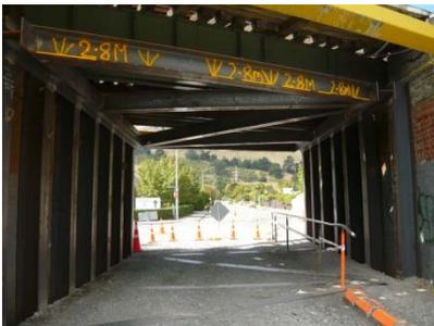
Fig 2 – Temporary repairs following earthquake
