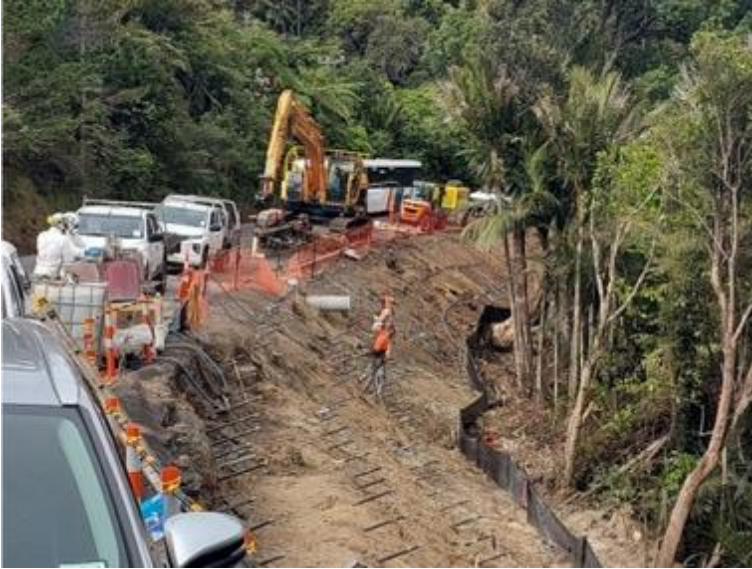
Wairere Road slip site 349 Wairere Road, left installing the soil nails, right – preparation for no fines concrete pour.
