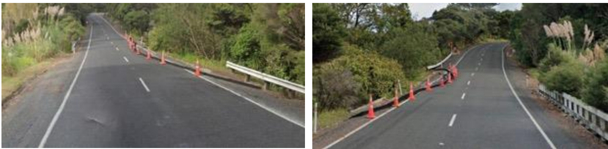
Site RP12.55, currently there are retaining walls on each side of the road, large upstream catchment and existing stream.
