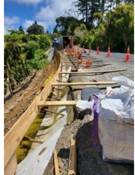
Wairere Road slip site 349 Wairere Road, left installing the soil nails, right – preparation for no fines concrete pour.
