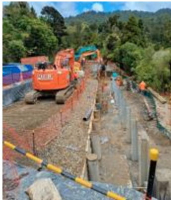
Scenic Drive RP6.73 site underway with installation of the retaining
