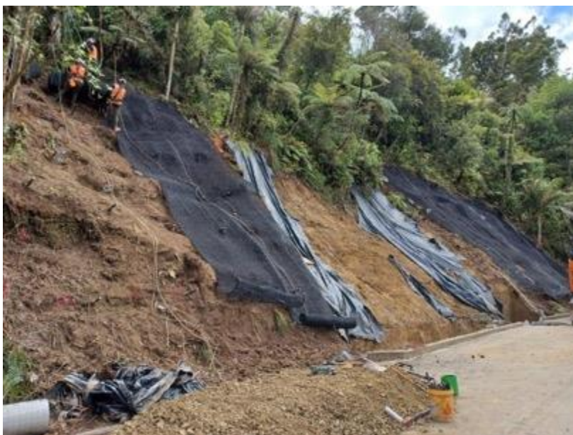
RP0.85 Scenic Drive Titirangi overslip has had soil nails installed, and the underslip has been retained with the backfill completed.
