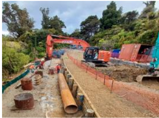
Scenic Drive RP6.73 site underway with installation of the retaining
