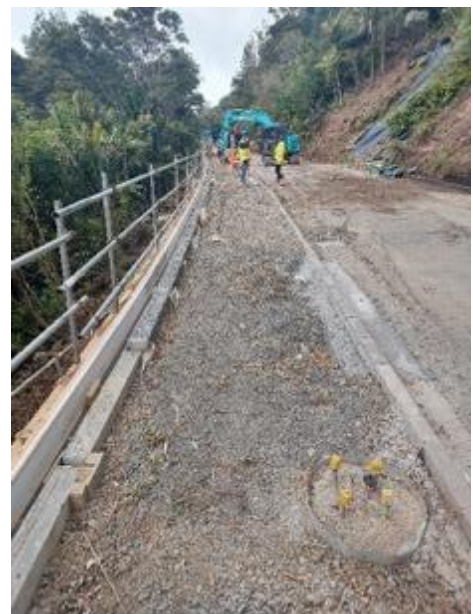
RP0.85 Scenic Drive Titirangi overslip has had soil nails installed, and the underslip has been retained with the backfill completed.
