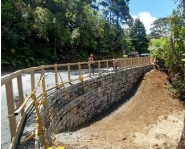
Slip site RPo.582 Karekare Road, installation of the rediblock wall and guardrail
