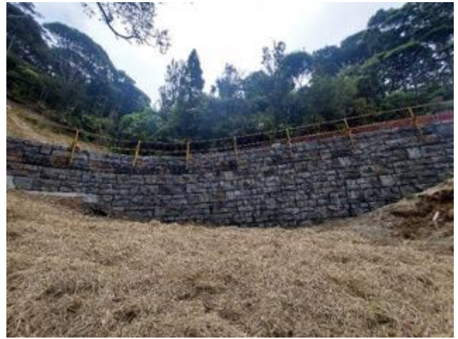
Slip site RPo.582 Karekare Road, installation of the rediblock wall and guardrail
