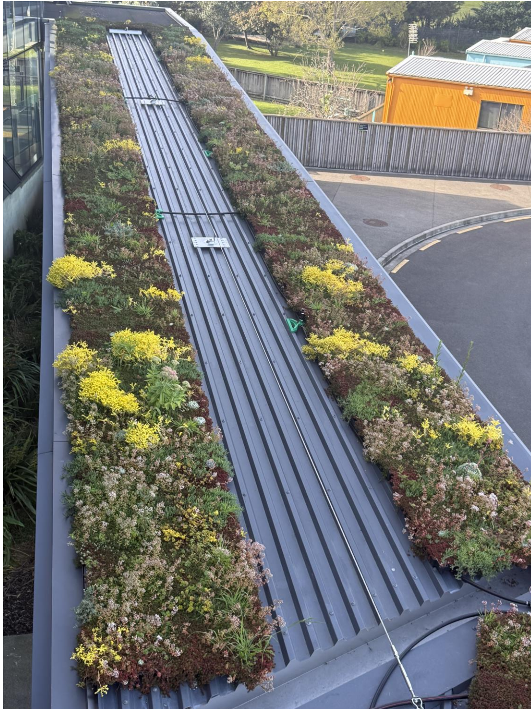
Figure 3: Green Roofs in Puhinui Station Bus Shelter
