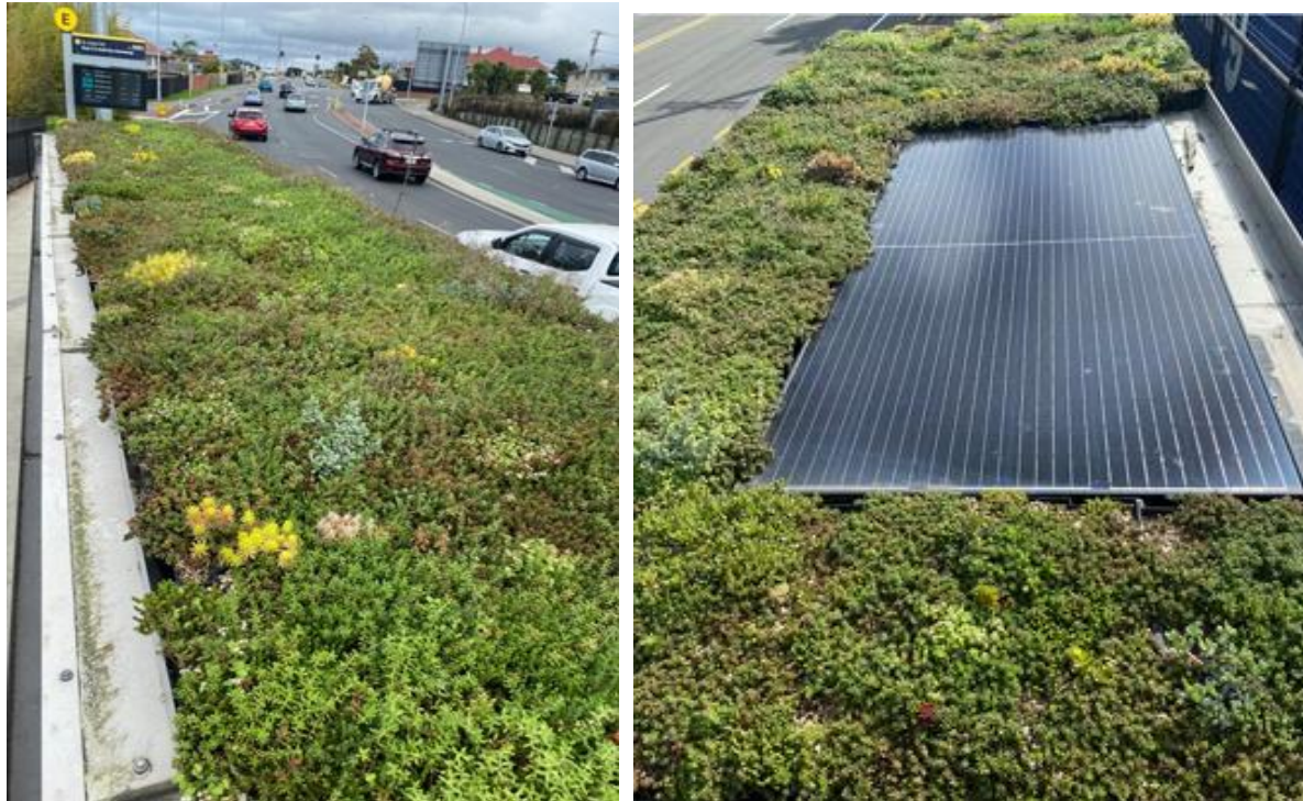
Figure 4: Green Roofs in Te Atatu Bus Shelter and (44 Portage Road, New Lynn)
