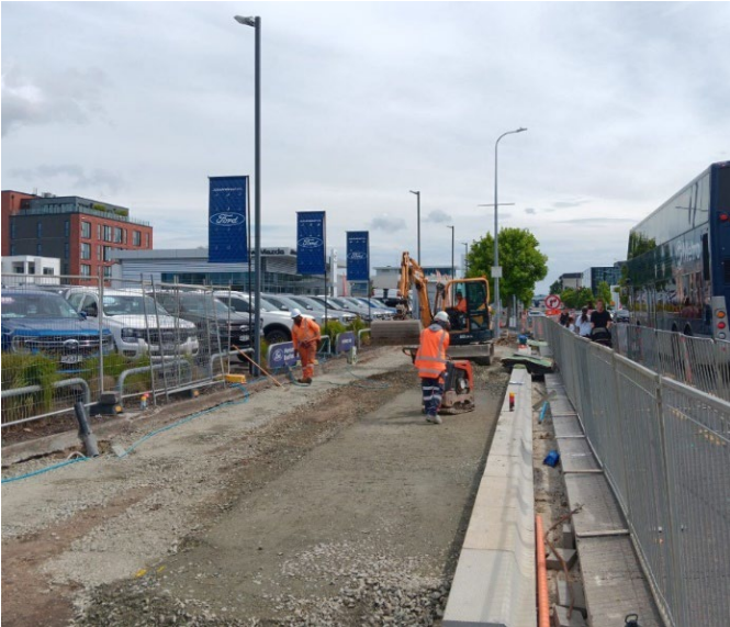
Building the bus platform near John Andrew Ford
